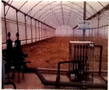
Figure 6. Irrigation system and nutrient mixer
