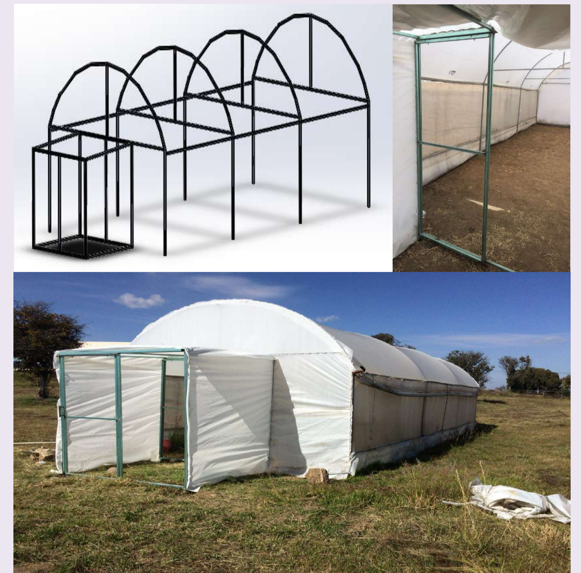
Figure 6 Profile of greenhouse structure, redesign in Solidworks.
